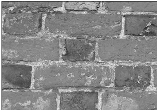
Brick pattern called Flemish Bond using burnt headers
